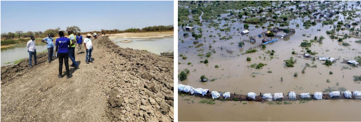
Figure 2.A: Lotilla makeshift River crossing point (temporarily backfilled river crossing points that connect two counties), B: Aerial view of section of Pibor town flooded
